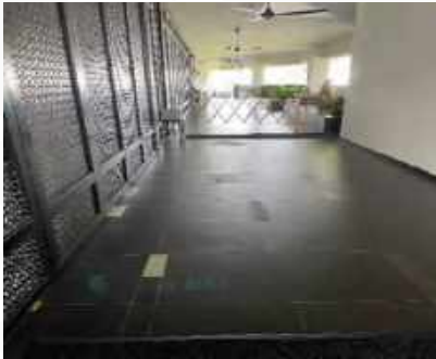
Zone A walkway to classes at level 3
